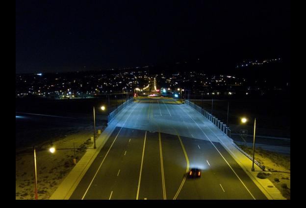
The even illumination of the overpass by ANP's high performance LED shows a sharp contrast to the roadway area leading up to the overpass.
