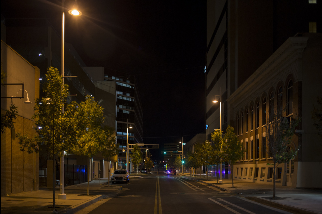
Before Retrofit (150-watt MH, 250-watt MH)
