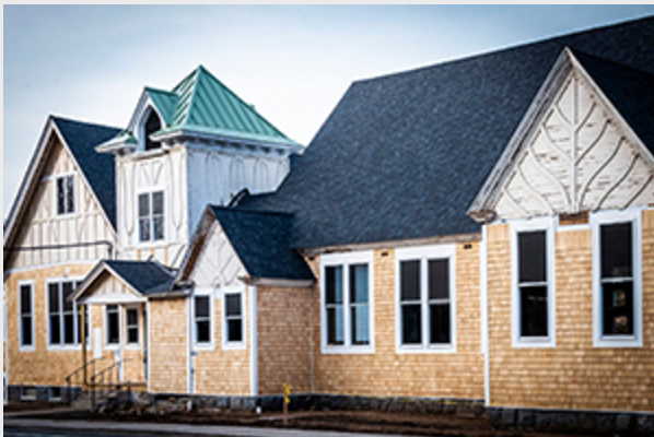
Renovation in Progress
