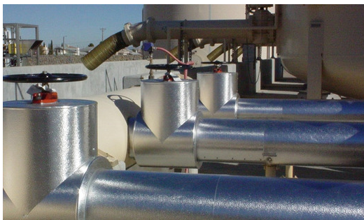
Insulation of pipes.
