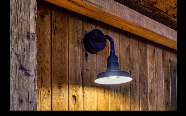
Solar power generates direct current to the battery storage system to power lighting, HVAC systems, security, audio and video systems. The system is DC, end to end, never converting to AC. ANP Lighting provided all fixtures with 24v DC input drivers to accept power from the facilities centralized system.
