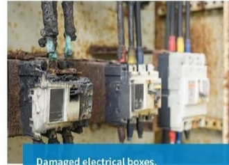
Damaged electrical boxes.
